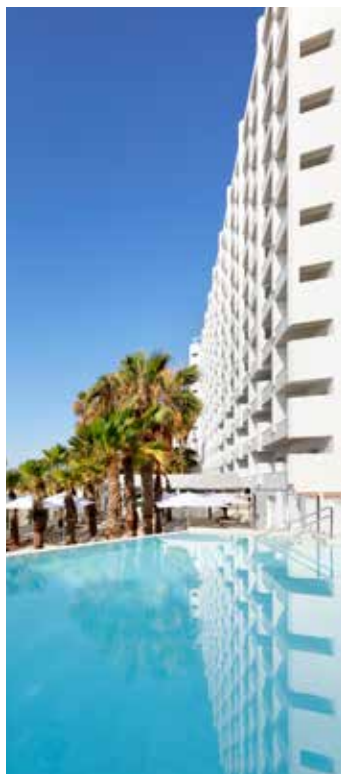
Palladium Hotel Costa del Sol, Spain
